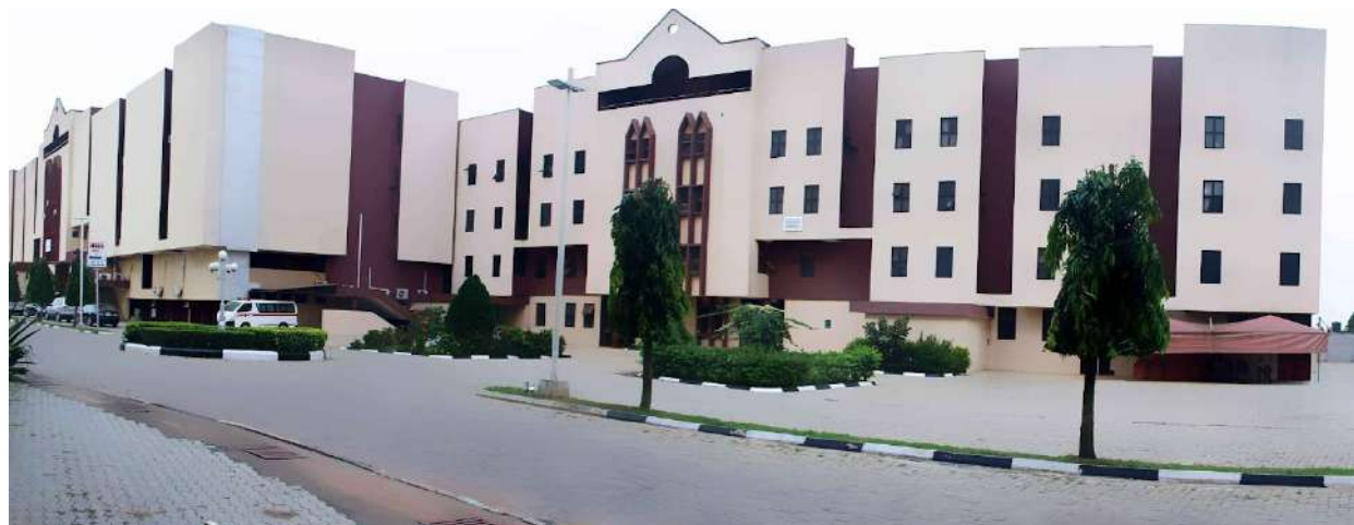
Wide view of Anchor University, Lagos campus showing the Admin building and a female hostel.
