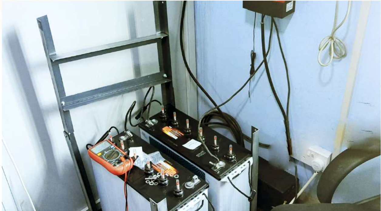
Installation of the inverter system at the AUL Space Lab.
